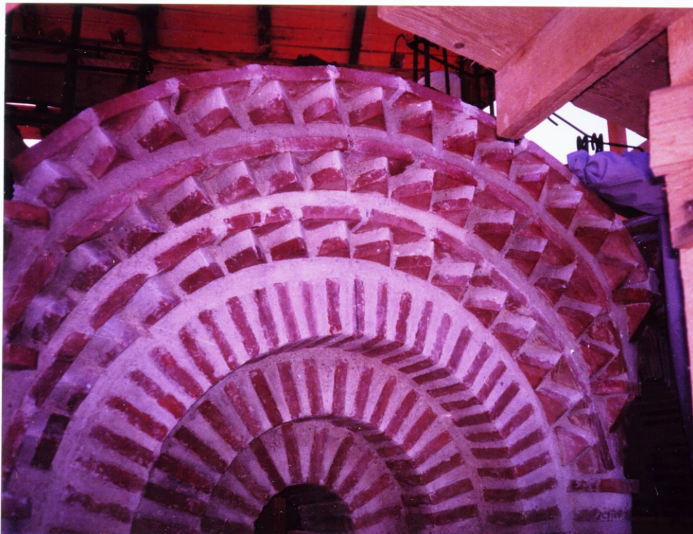
Fig. 5: Plataresti, arcade above drum in construction
