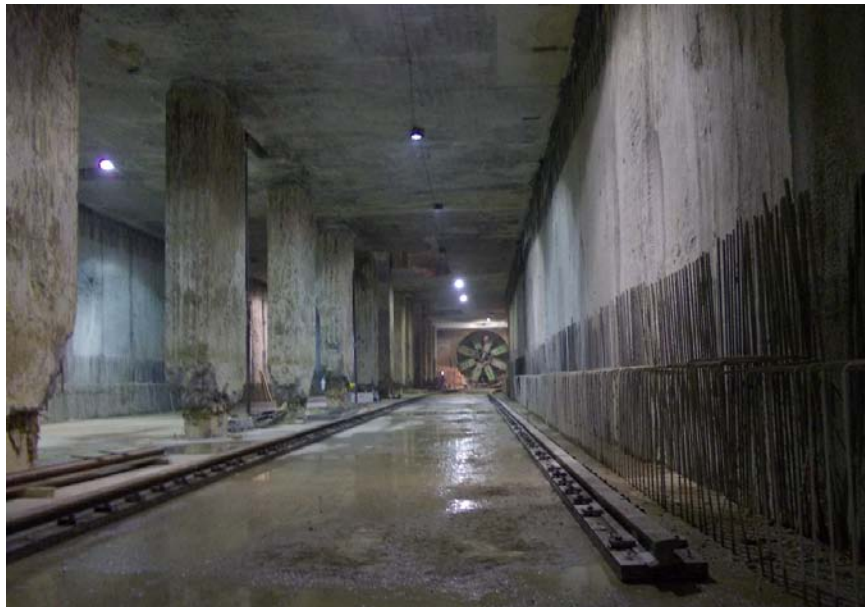
“Fig.2 Execution of molded walls in subway stations”
